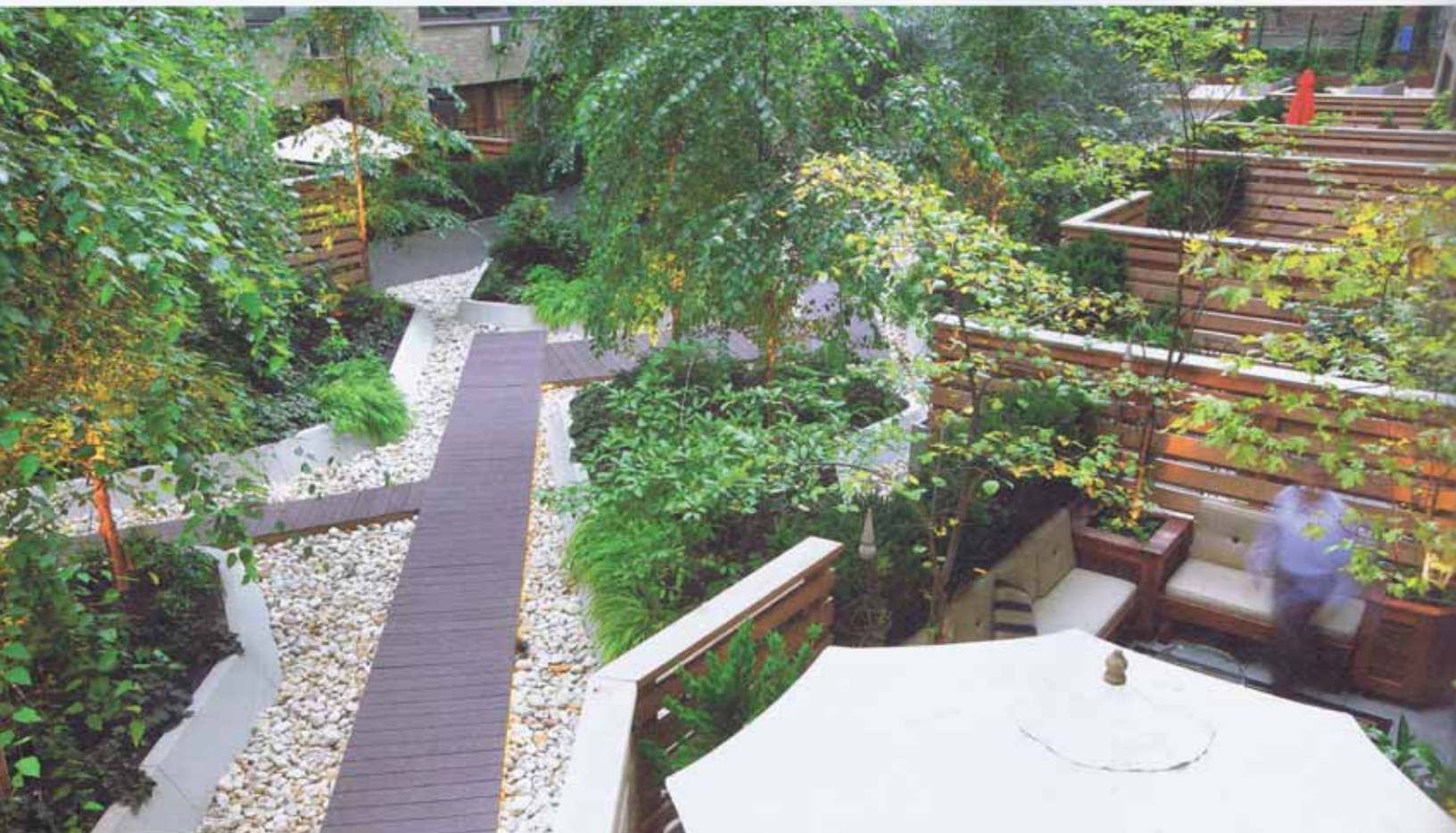
The solution for the garden in Chelsea Lane is a modular curb system that forms sinuously curving large planting areas that can support large soil volumes.
